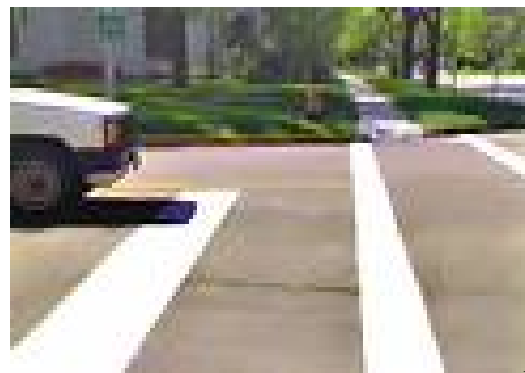
Intersection stop lines
